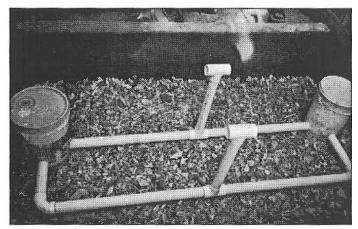
This photo shows a small wastewater garden that also handles sink water. The drywall buckets hold nylon filters, which can be replaced and cleaned. The pipe risers add aeration to boost performance.
