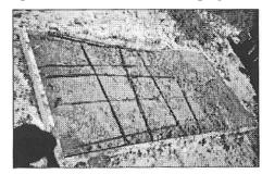
Packing the base slab with cement and laying rebar reinforcement.
