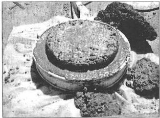
The sawed-off top of the bucket makes a good mold for the lid for the inactive toilet riser. Insert a bent rebar handle on the top. (This is dug into the ground.)
